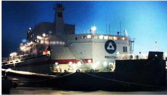
The Akademik Lomonosov floating nuclear power plant (Image: Rosatom)
